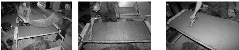
Figure 5. Mounting of the TRC strengthening system. Courtesy of A. Brueckner, Dresden University of Technology.
