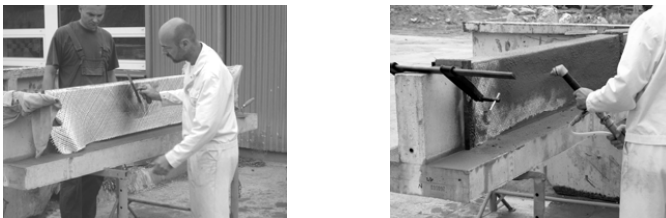
Figure 3. Mounting of the TRC strengthening system. To the left, the fabric is laminated onto the side of the beam. To the right, a layer of cement matrix is sprayed on to the surface of the fabric. Courtesy of A. Brueckner, Dresden University of Technology.
