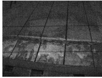
Slab and beam geometry and markings prior to the sawing of the beams with the carbon fiber grid cut at the ends of the mortar
