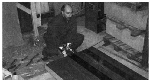
Fig. 4. Bonding the CFRP fabric to Slab 5
